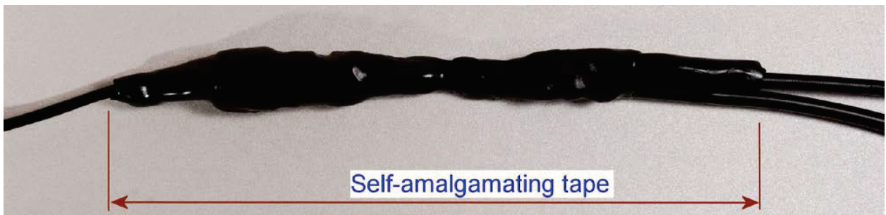
Figure 104 Wrapping self-amalgamating tape around the GPS adapter cable joint
